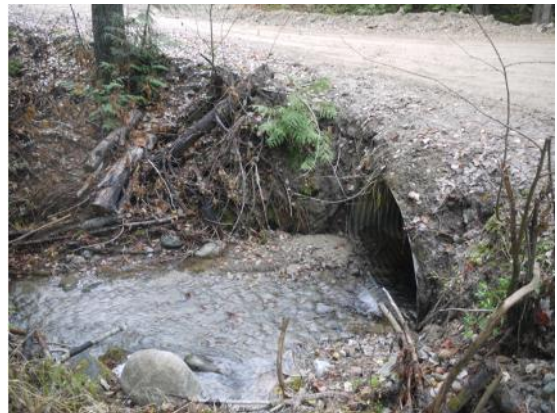
Figure 2. Example of resource road crossing a small stream. Note sediment over and adjacent culvert (J. Coleshill photo).
